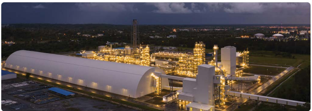
The BFI Plant is Brunei's premier ammonia and urea plant with a production nameplate capacity of 2,200 metric tons of ammonia per day, which is converted to produce 3,900 metric tons of granular urea per day.
