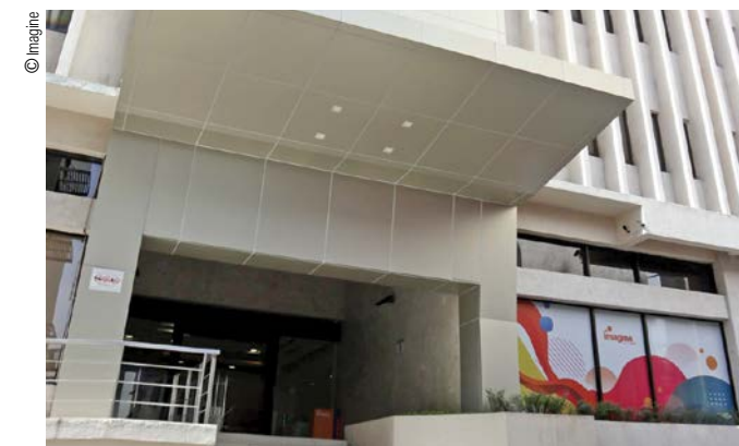
The headquarters of Imagine, one of Brunei's leading digital services companies
