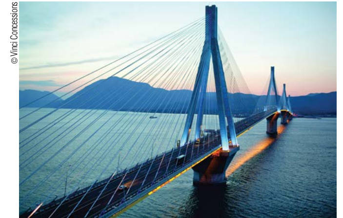
© Vinci Concessions Vinci Concessions "Charilaos Trikoupis" Bridge (Rio-Antirrio straits)
