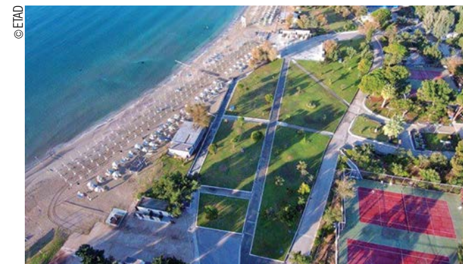
ETAD's portfolio ranges from hospitality assets to office buildings and land plots
