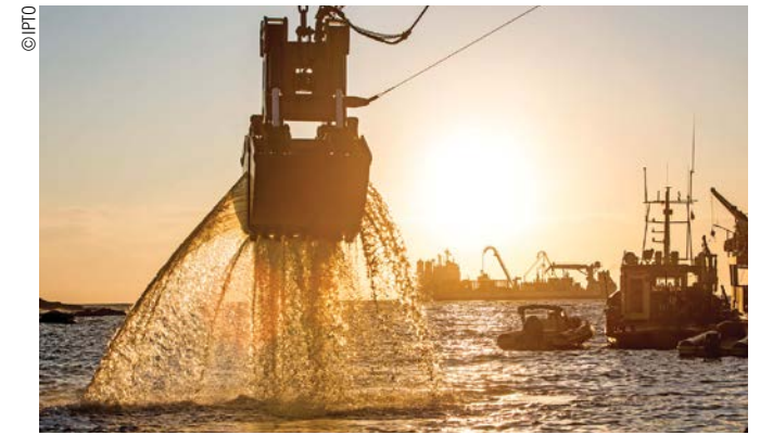
IPTO's underwater laying activities around the islands
