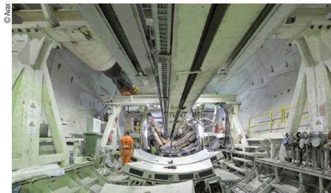
Construction works are on for the Athens Metro extension
