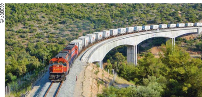
An extended maintenance program for rolling stock will boost rail services
