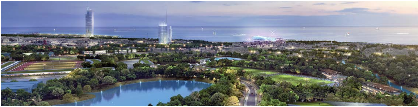
Lamda Development's landmark Hellinikon project
