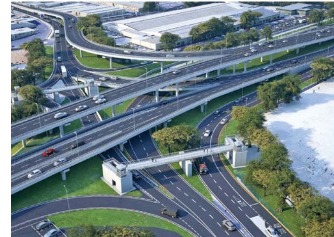
The government has committed itself to major road infrastructure projects
