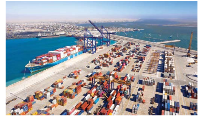
Namport's new terminal at the Port of Walvis Bay doubles its container capacity
